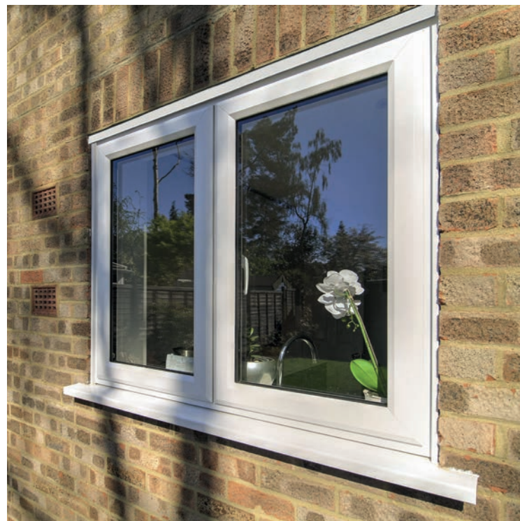
Concealed Ventilation installed through the outer frame
