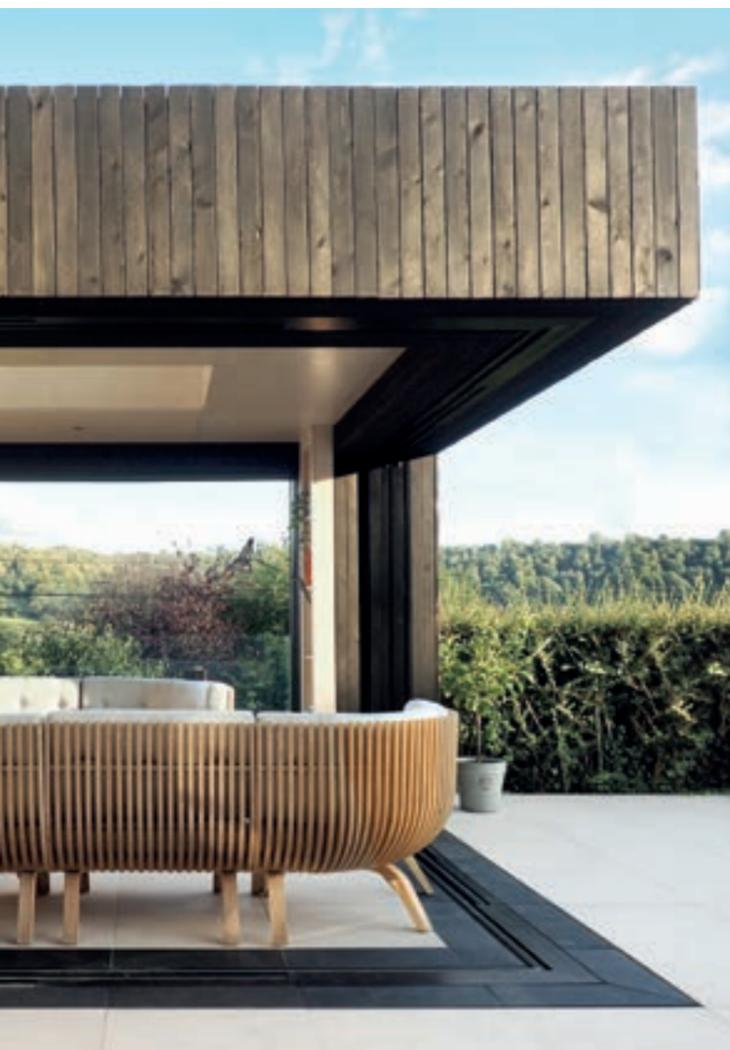
Created with an integrated corner post, our floating corner sliding doors can be slid back to create a completely open corner that allows your home to connect with your garden to create the appearance of a room that never ends.
