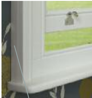
Normal Replacement Box Sash may project into the room.
